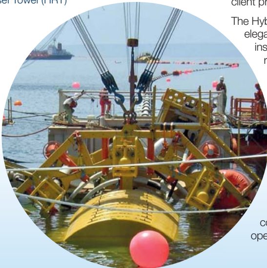
Preparing to install a Hybrid Riser Tower (HRT)
